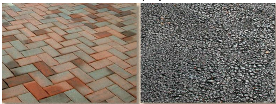
Figure 13. Some types of permeable pavement.
